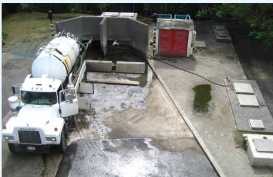
Figure 9.10 Faecal sludge discharge at Illidge Road wastewater treatment plant at the buffer tank.
