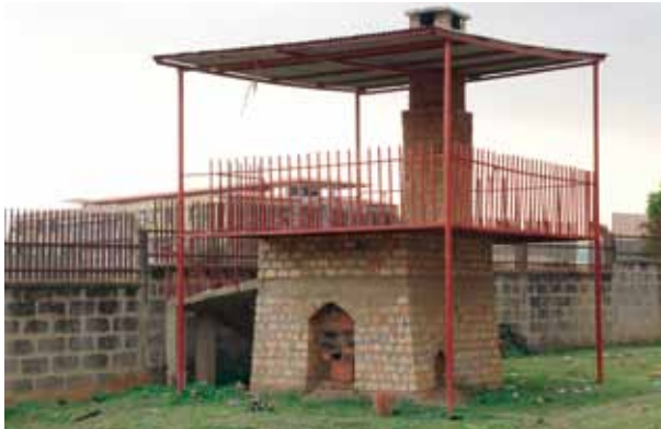
Figure 18.6 FaME (Faecal Management Enterprises) project pilot scale kiln for co-combustion of faecal sludge in brick production in Kampala, Uganda (photo: Pitman Ian Tushemeziwe).
