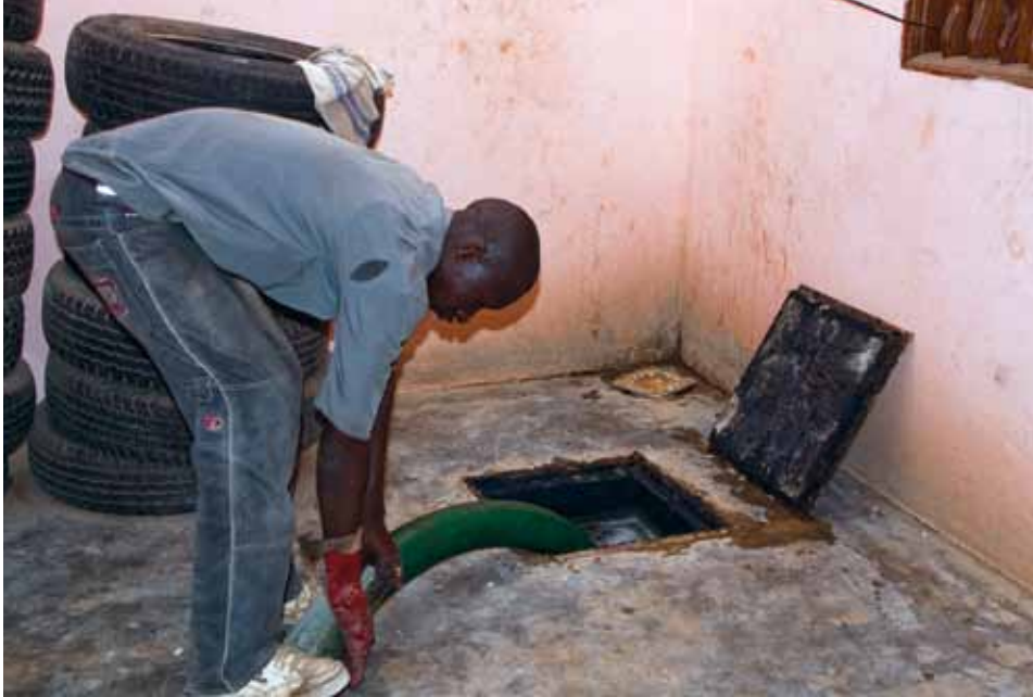
Figure 4.2 An example of an emptying operation in Dakar, Senegal where the system is located in an internal courtyard and gaining access requires cooperation with the residents (photo: Linda Strande).
