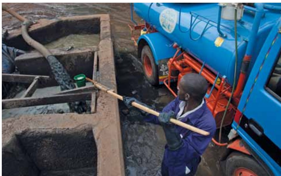
Figure 18.3 Implementation of the FAQ method (Faecal Sludge Quantification and Characterisation) in Kamapla, Uganda (photo: Lars Schoebitz).
